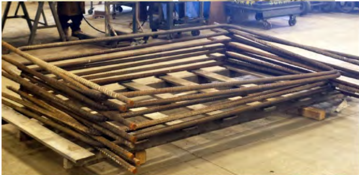
Rebar Fabrication up to 1 ½" Diameter Rebar
